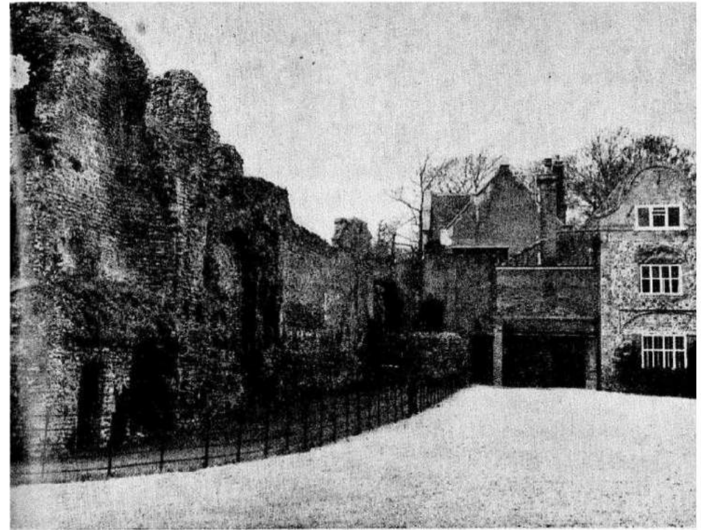
Side and rear of Claxton Castle looking north-west.
